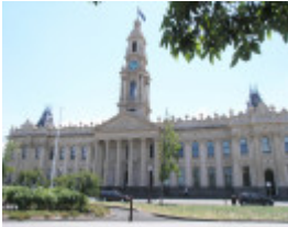
SOUTH MELBOURNE TOWN HALL SOHE 2008
