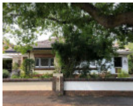
2B-2C Coppin Street, Malvern East
