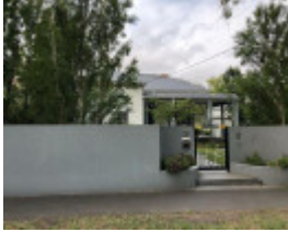
18 Coppin Street, Malvern East
