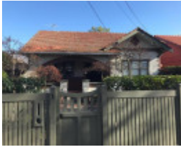
1 Turner Street, Malvern East
