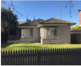
2 Turner Street, Malvern East
