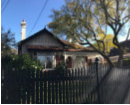
5 Turner Street, Malvern East
