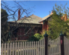
8 Turner Street, Malvern East
