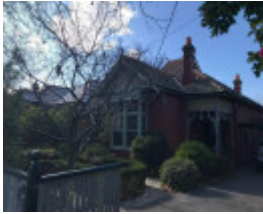
10 Turner Street, Malvern East
