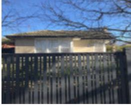
13 Turner Street, Malvern East
