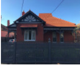
18 Turner Street, Malvern East
