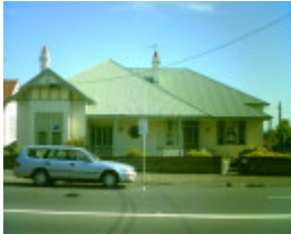
10 Aberdeen Street, Geelong West
