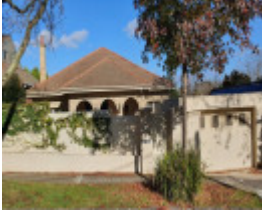
2 Stradbroke avenue, TOORAK
