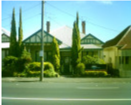
14 Aberdeen Street, Geelong West
