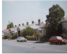
Source: Aitken, Honman & Huddle, 'City of Geelong West Urban Conservation Study', 1986. - Street View
