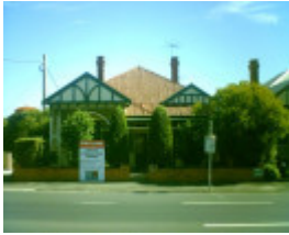
18 Aberdeen Street, Geelong West
