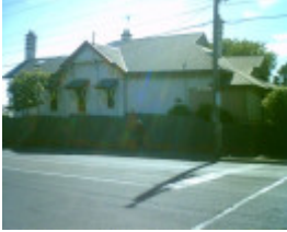
62 Aberdeen Street 1, Geelong West
