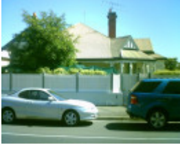
68 Aberdeen Street, Geelong West
