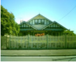
78 Aberdeen Street, Geelong West
