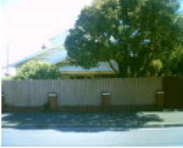
86 Aberdeen Street, Geelong West
