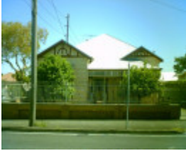
90 Aberdeen Street, Geelong West
