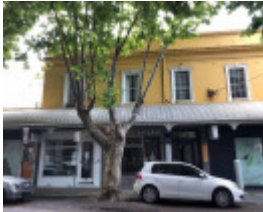
81 Davis Avenue, South Yarra
