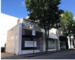
41 Ralston Street, South Yarra
