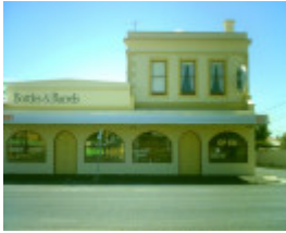
132 Aberdeen Street, Geelong West
