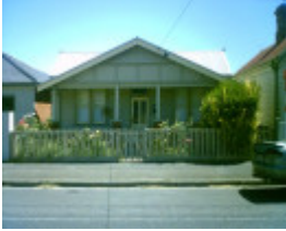
152 Aberdeen Street, Geelong West
