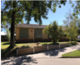
1 Oravel Avenue, Malvern East
