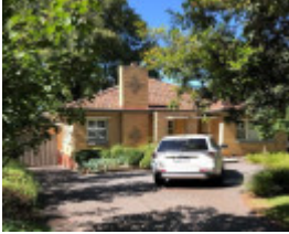
6 Oravel Avenue, Malvern East
