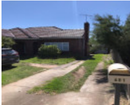
481 Waverley Road, Malvern East
