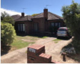
483 Waverley Road, Malvern East
