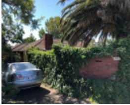
487 Waverley Road, Malvern East
