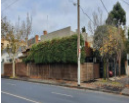
1-6 St Malo Street, Prahran
