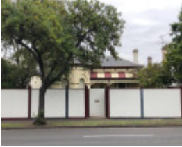
75 Williams Road, Windsor
