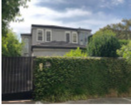
6 Henderson Avenue, Malvern
