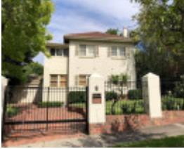
7 Henderson Avenue, Malvern
