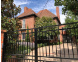
15 Henderson Avenue, Malvern
