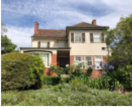
19 Henderson Avenue, Malvern
