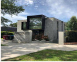
14 Robinson Street, Malvern
