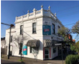
1 Claremont Avenue, Malvern
