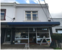
5 Claremont Avenue, Malvern
