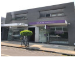
19-21 Claremont Avenue, Malvern
