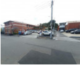
2-6 Llaneast Street, Armadale
