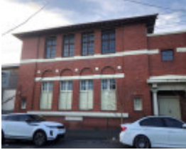
8-10 Llaneast Street, Armadale
