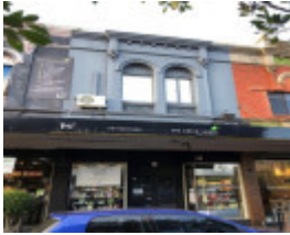
9 Station Street, Malvern
