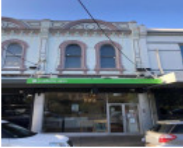
33 Station Street, Malvern
