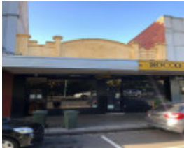
41-43 Station Street, Malvern
