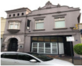
49 Station Street, Malvern
