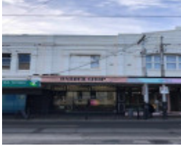
115 Wattletree Road, Malvern
