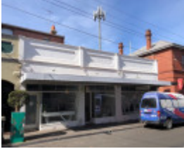
2A Willis Street, Armadale
