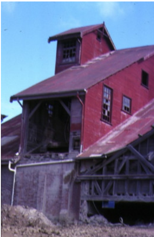
former standard brickworks federation street box hill red corrugated iron building
