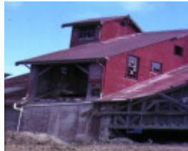
former standard brickworks federation street box hill red corrugated iron building
