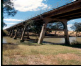
h01986 janevale bridge from sw jan02
