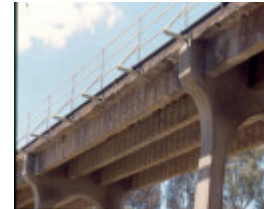
H01986 janevale bridge from sw girders jan02
