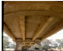
H01986 janevale bridge underside from s jan02
