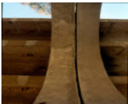
H01986 janevale bridge underside expansion joint jan02
