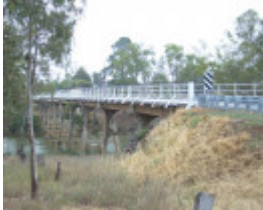
JANEVALE BRIDGE OVER THE LODDON RIVER SOHE 2008
