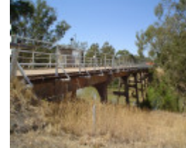
h01986 1 janevale bridge over loddon river laanecoorie deck she project 2004
