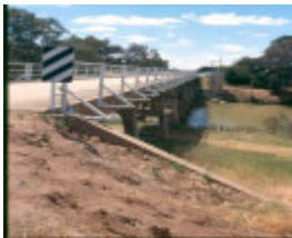
H01986 janevale bridge deck from s jan02
