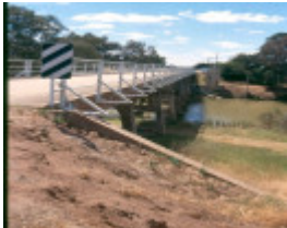
H01986 janevale bridge deck from s jan02
