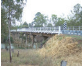
JANEVALE BRIDGE OVER THE LODDON RIVER SOHE 2008
