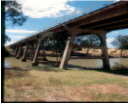
h01986 janevale bridge from sw jan02
