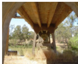
h01986 janevale bridge over loddon river laanecoorie close up underneath she project 2004
