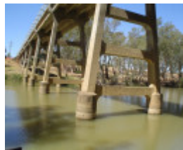
h01986 janevale bridge over loddon river laanecoorie base she project 2004
