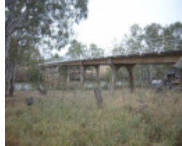
JANEVALE BRIDGE OVER THE LODDON RIVER SOHE 2008
