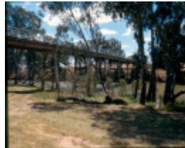
H01986 janevale bridge from se jan02
