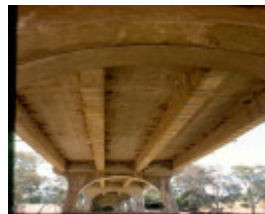
H01986 janevale bridge underside from s jan02
