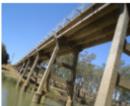
h01986 janevale bridge over loddon river laanecoorie beneath she project 2004
