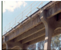
H01986 janevale bridge from sw girders jan02
