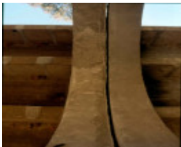
H01986 janevale bridge underside expansion joint jan02
