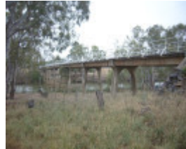
JANEVALE BRIDGE OVER THE LODDON RIVER SOHE 2008
