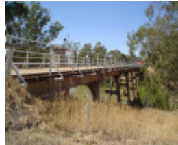
h01986 1 janevale bridge over loddon river laanecoorie deck she project 2004
