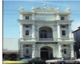
1 former colonial bank bendigo front view dec1993
