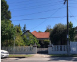
427 Wattletree Road, Malvern East
